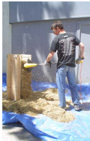
(b) Trimming bale in jig.
